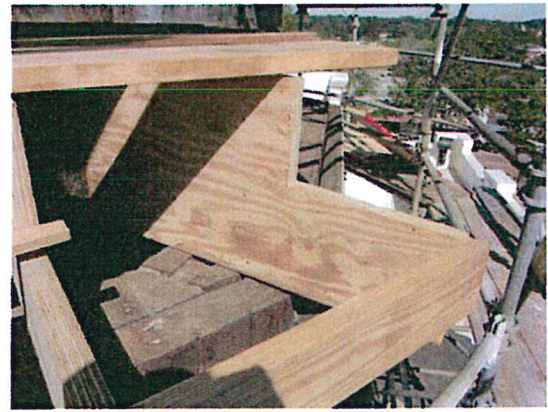
Figure 10 –Stepped Outrigger Installation
