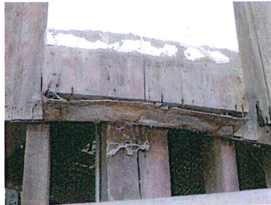
Figure 12 – Wood Pilaster Cut-In for Flashing
