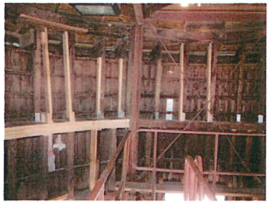
Figure 16 –Interior Structural Repairs
