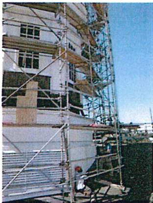
Figure 17 – Cupola Base Preparations
