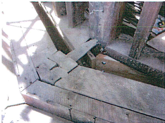
Figure 9 – Original Beam/Column Joinery Detailing
