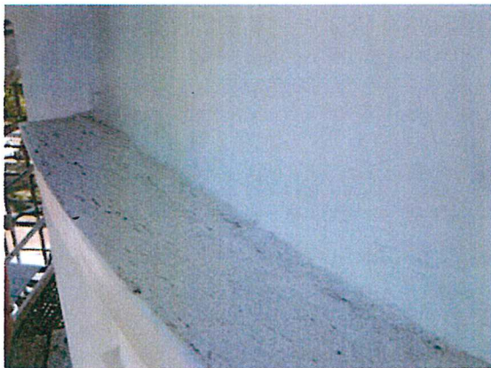
Figure 11 – Window "Eyebrow" Flashing
