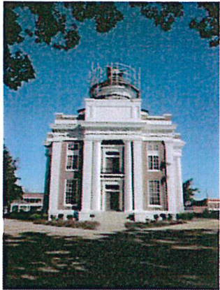
Figure 1 – South Elevation with Scaffolding at Cupola
